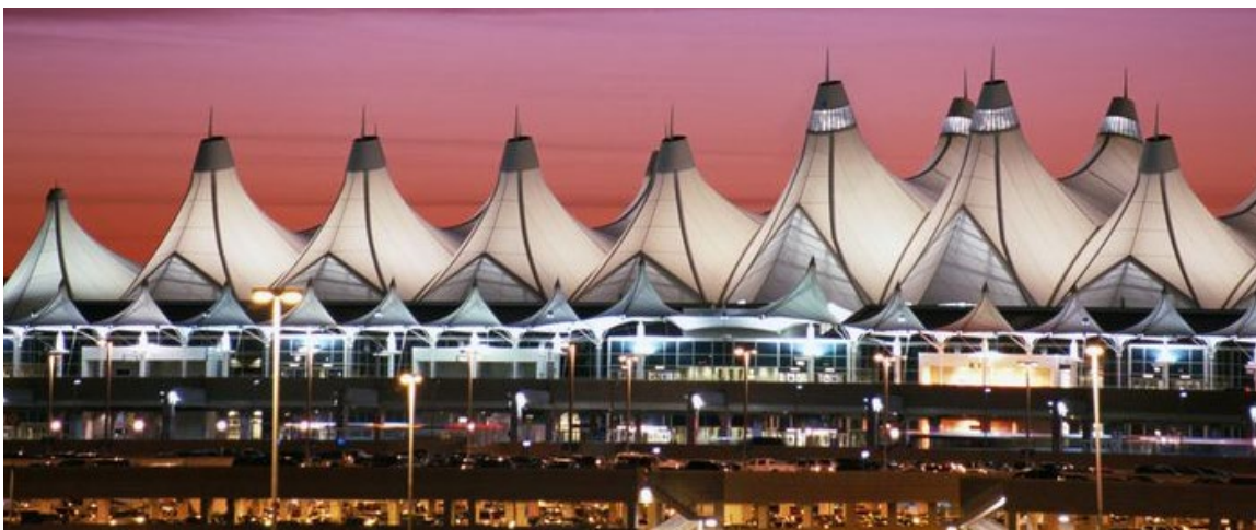
Figure 7. A section of the Denver International Airport showing the tent-inspired roof (Madere 2016).
