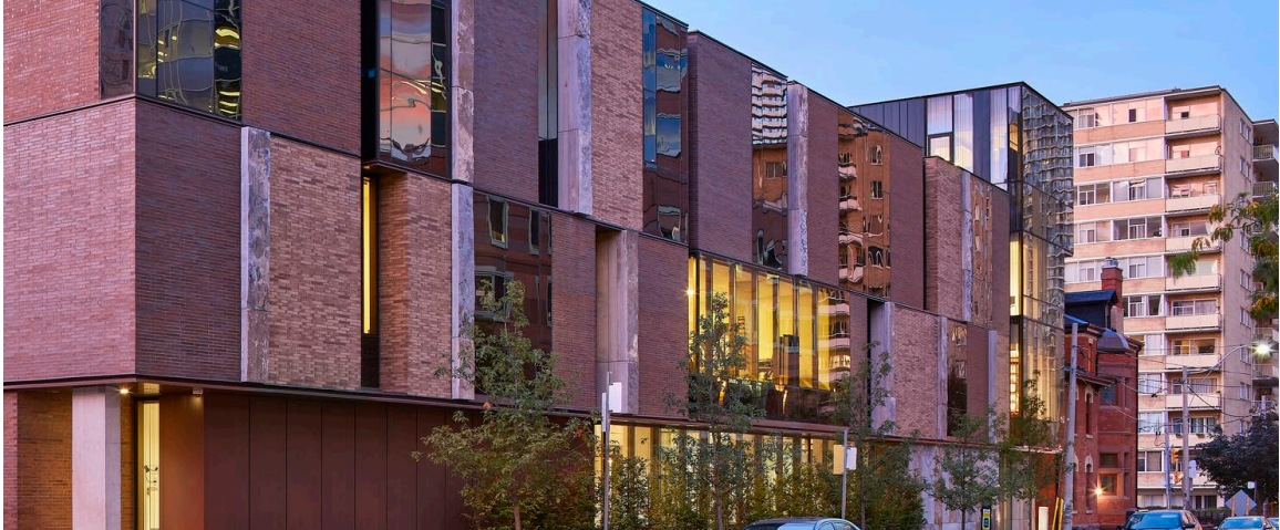
The addition to Casey Hall draws inspiration from the AIDS quilt using different materials like different pieces of fabric. Photo by Doublespace Photography, 2017 (Hariri Pontarini Architects 2018).
