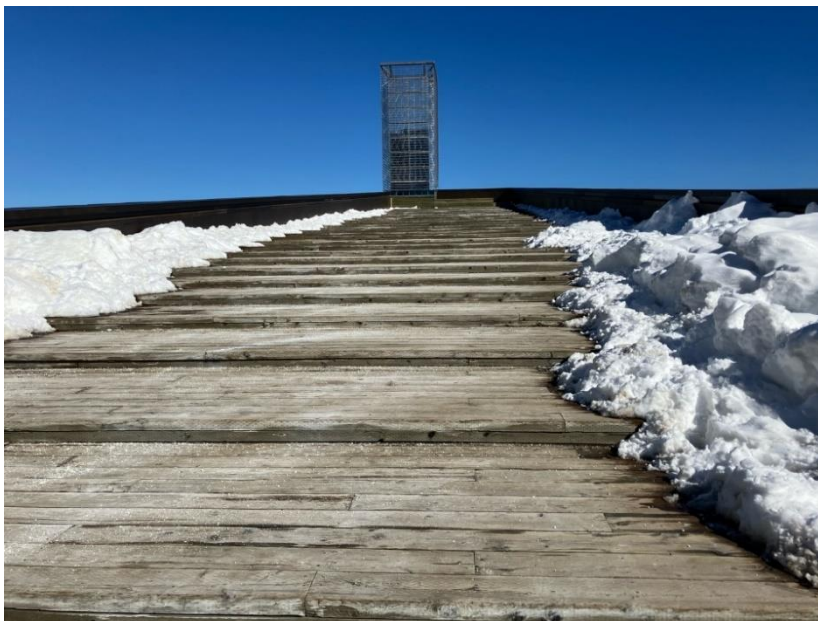
Figure 5.6: Upward Staircase of the QM
