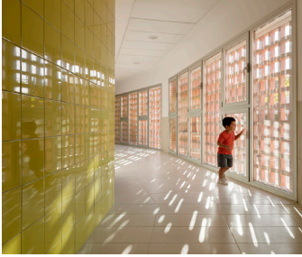
Figure 51: This image shows the use of parametric walls that control light and perception and provides a sense of privacy and exploration (Villalba 2021).
