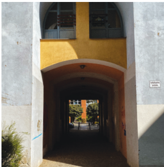
Portals and arcades of the internal streets and courtyards at Ritterstrasse, Berlin.
