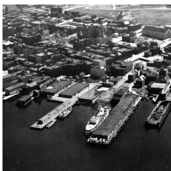
Downtown Halifax before many of the demolitions in the Central Redevelopment Area. (HMA 1961)
