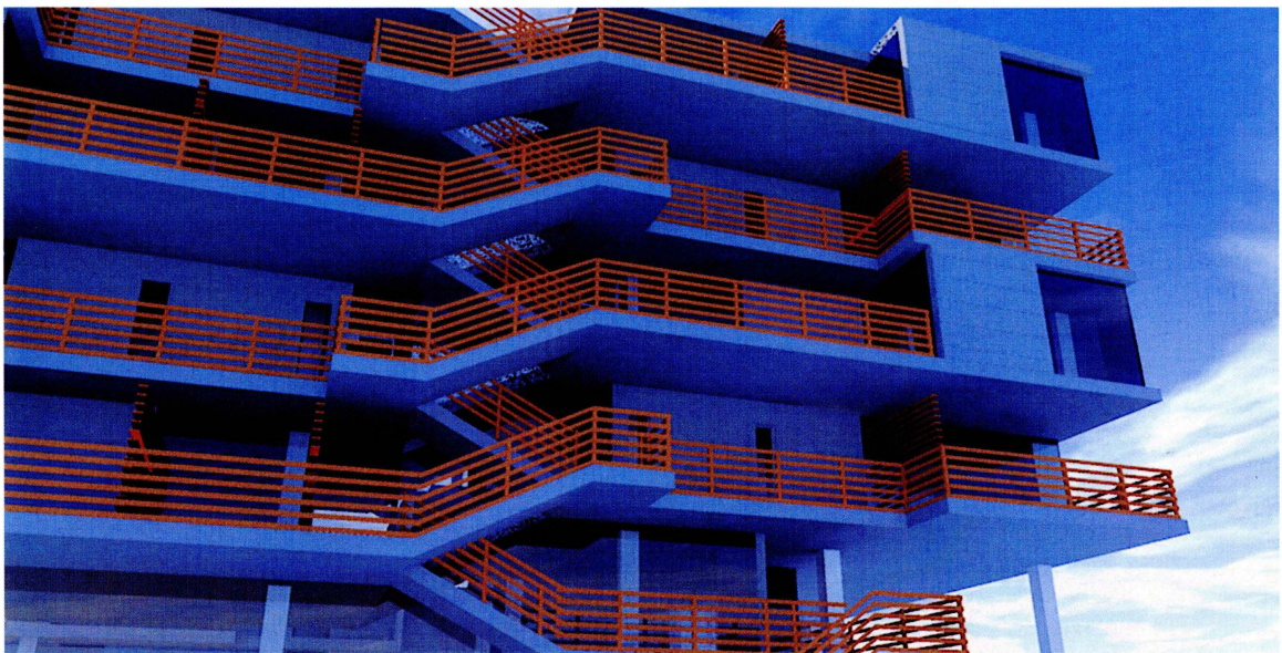
Balconies linked by external stair.
