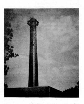
Above photo shows the Sanatorium 'stack with the finishing touches on the recent retopping. It is 115 feet high and 5 feet in diameter at the top. Material, red radial brick.
