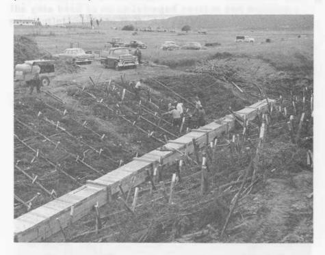
Fig. 10 - Abt. #1 on Allan River Marsh, Anna. Co.,  $\overline{\text{N.S.}}$ , under construction. The sluice has been set on its bed, and brushing of the aboiteau fill is in progress. Brushing, as shown here, is done between every 2 ft. layer of fill. (Photo N.S. 30//10)
