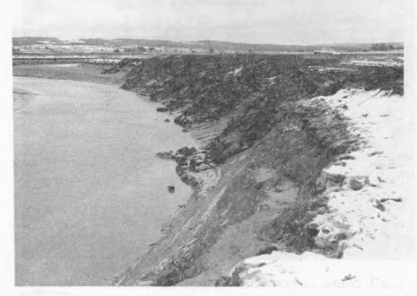
Fig. 8 - The same view as in the above photograph; after heavy rock has been placed over the bank in a series of piers. This method proved to be the most permanent protection against undercutting. (Photo 21-054).
