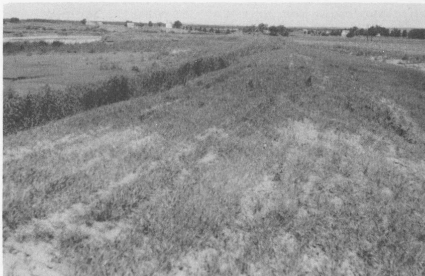
Fig. 3 - The inside slope of a dyke constructed in 1950 with grass sown early in 1951. This photograph was taken in August of 1951.
