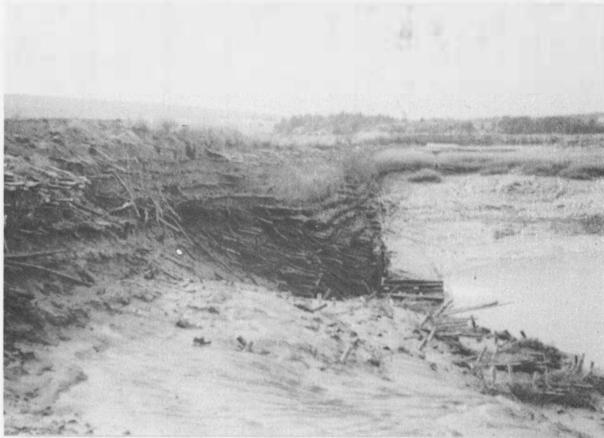
Fig. 7 - The sea-side of a large aboiteau in Albert County, N. B. Note how the tide water has removed the earth fill from between the brush layers. In the immediate foreground is temporary brush work as a means of repairing the weakest spot in the fill while a new structure was being erected.
