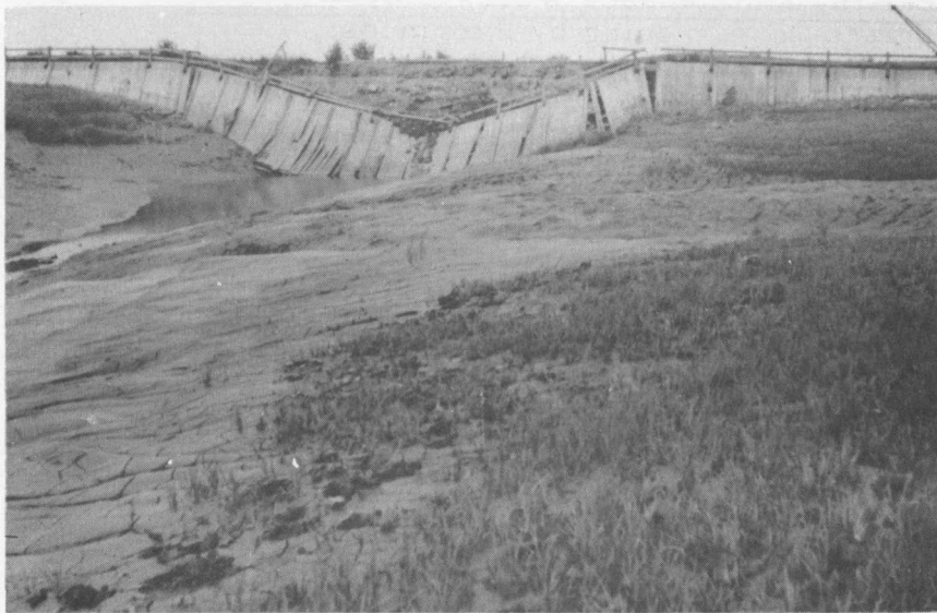
Fig. 11 - This structure is a combined aboiteau and highway crossing near Belliveau Village, N. B. The sluice was worn to a considerable degree and the entire facing on the sea-side of the structure has broken away. New Brunswick aboiteaux are being constructed with a slope of 3-1, and in the case of the larger structures a gravel facing is being placed.
