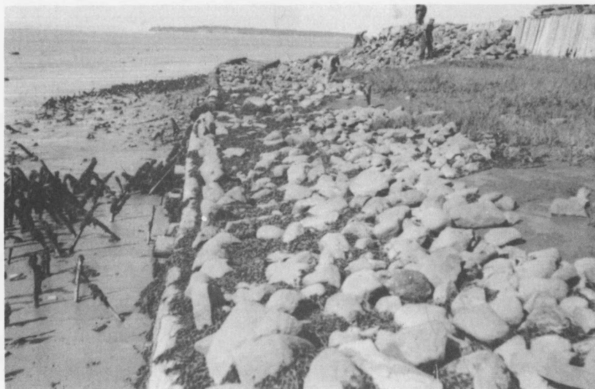
Fig. 17 - A view of old rock crib work being repaired in the vicinity of Annapolis Royal, N.S. At extremely vulnerable points this type of protection is required to prevent under-cutting of the dyke.
