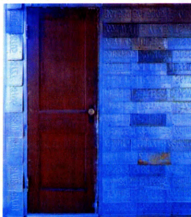
Re-use of waste material: car plates. Photograph of Cardboard Pod by Timothy Hursley, Alabama (2001). Rural Studio, Samuel Mockbee and an Architecture of Decency , 83.
