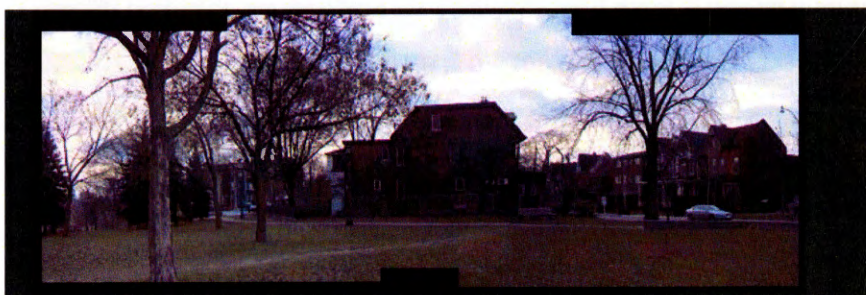
Site 7: Residential Street Condition (Crawford Street)
