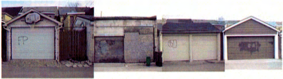
Photograph of garages along laneway (Site No.5)
