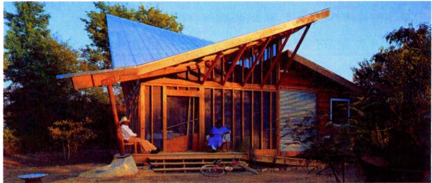
Front porch of Harris residence. Photograph of Harris Butterfly House (1996-1997). Rural Studio, Samuel Mockbee and an Architecture of Decency , 32.
