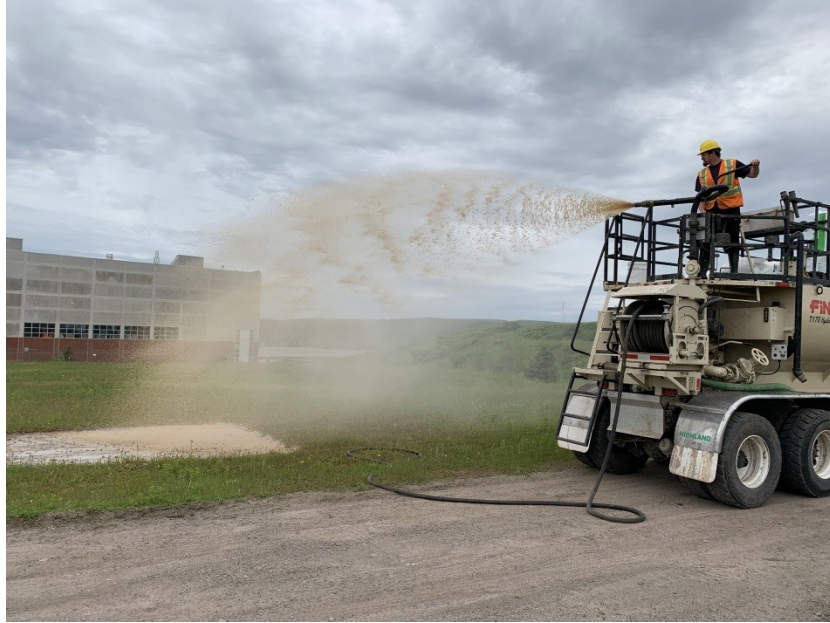
Figure 37 - Cannon style spraying technique to cover large areas and avoid clogging of larger particles. Spray contained grass growth composed of 40% Creeping Red Fescue ( Festuca rubra ), 30% Perennial Ryegrass ( Lolium perenne ), and 30% Kentucky Bluegrass ( Poa pratensis ).
