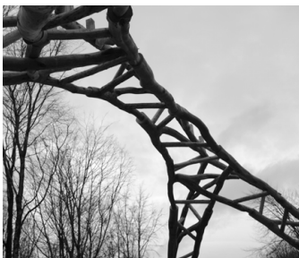
Fig. 25. The Tree Fork Truss
