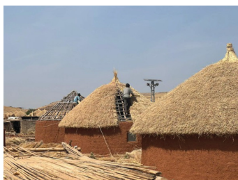
Traditional quttiyah or tukkul construction in Eastern Sudan. (Norwegian Refugee Council 2022)
