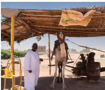
Owner of a traditional sesame press poses under his rakubah. Traditionally, even the posts of the rakubah would be of large branches, but in this instance steel posts are used.
