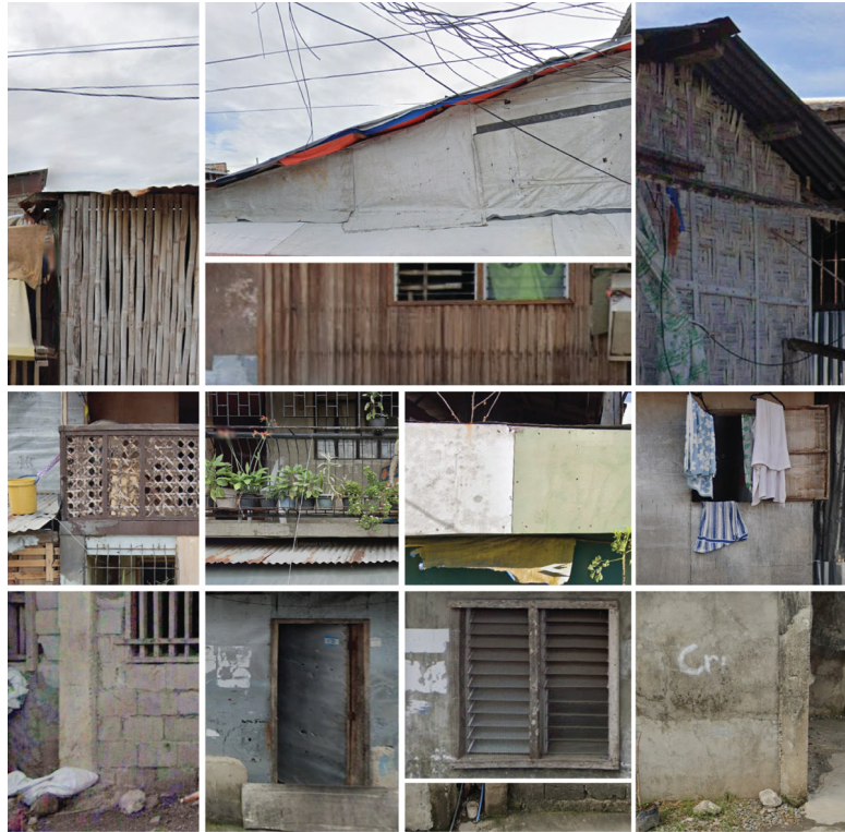
Materials used in Barangay 37, a “Makeshift-Dwelling” settlement in Tacloban City (GoogleEarth 2022)
