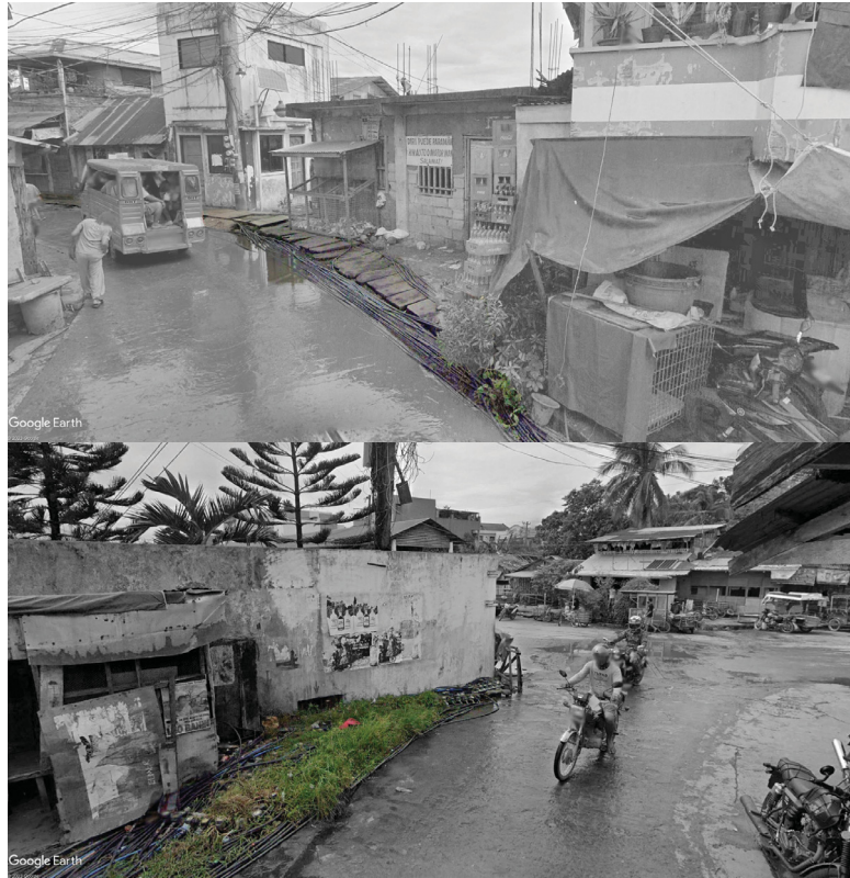
Inadequate sewage and water line in Barangay 37, Tacloban City, (GoogleEarth 2023)
