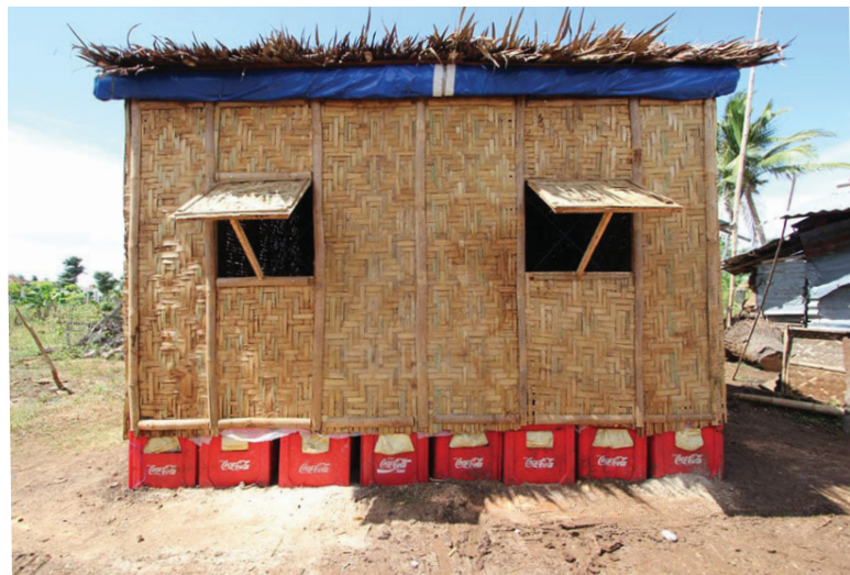
Shigeru Ban constructs his Paper Log House in Cebu, Philippines, after typhoon Haiyan (Shigeru Ban Architects 2014)
