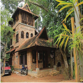
Exterior view of the house made from salvaged materials and brick in Kerala. (Ravi 2020)
