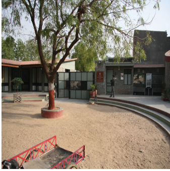
Courtyard view of the Manav Sadhna activity centre which is made using salvaged waste materials. (Pandya 2011)
