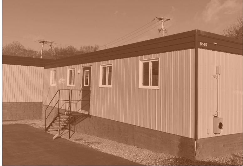
Dartmouth supported housing facility. Photograph by Ethan Lycan-Lang and Leslie Amminson. (Lycan-Lang and Amminson 2022)
