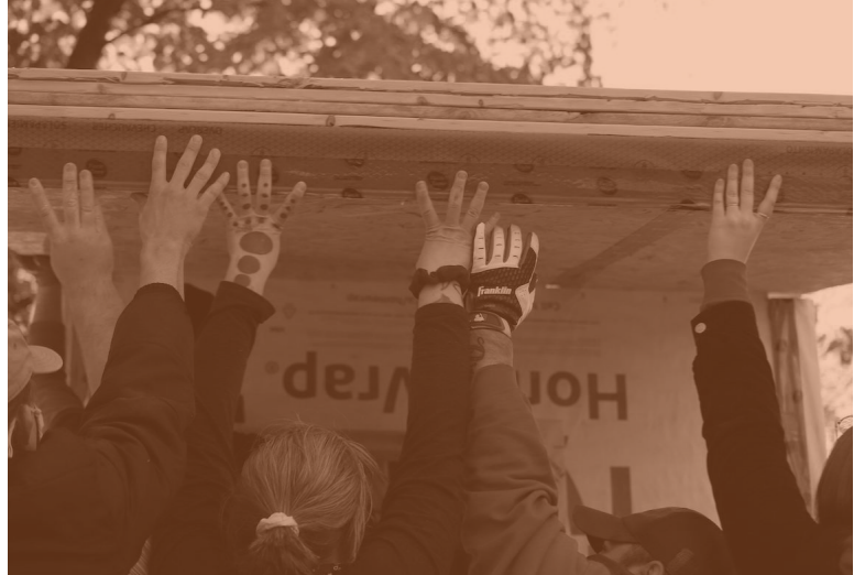
Halifax Mutual Aid crisis shelter construction. Photograph by The Coast . (Walton 2021a)
