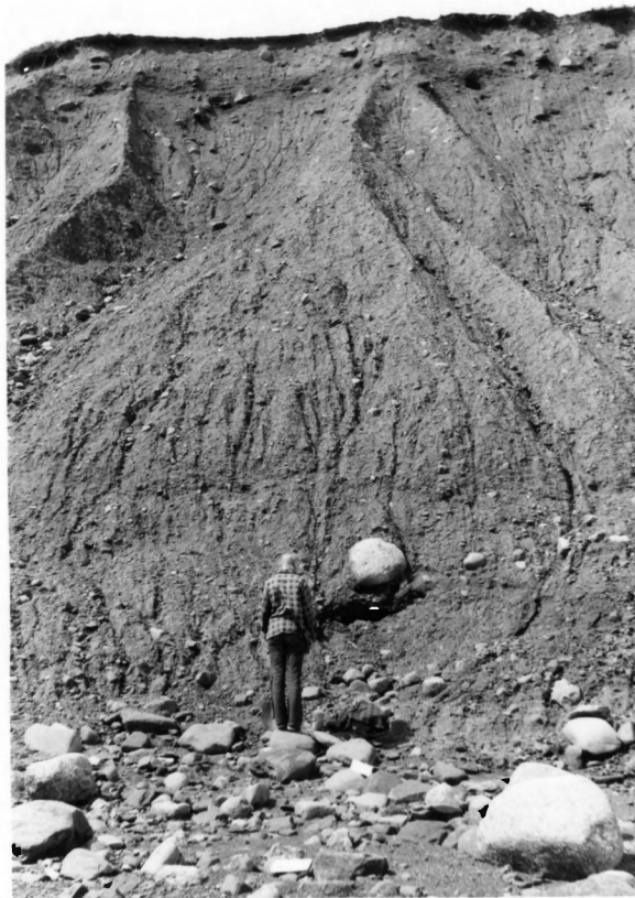
Extensive gullying and boulder armour.
