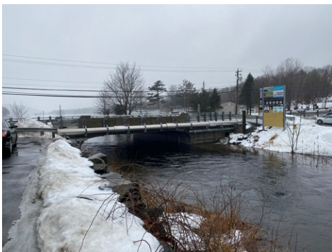
Figure 34: Location A - Bridge showing high water
