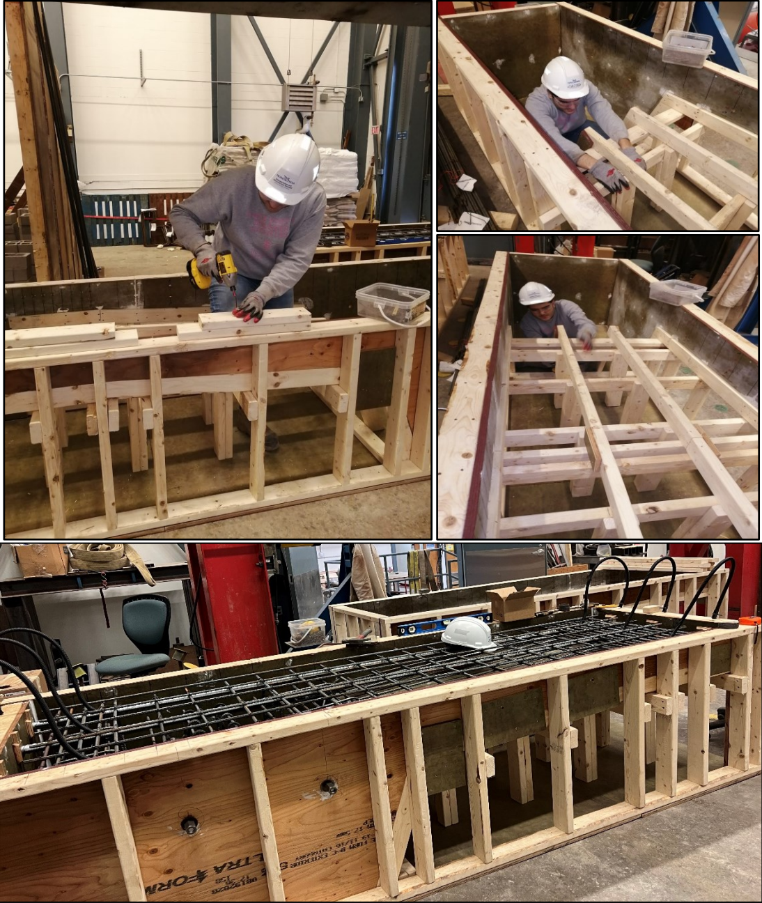
Figure 4-5. Bridge Cantilever Specimen Fabrication
