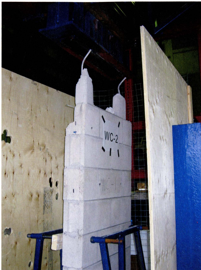
Figure 4.15 Failure mode of wall specimen WC-2
