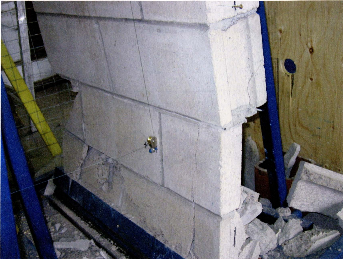
Figure 4.17 Crushing of compressive face in WC-3
