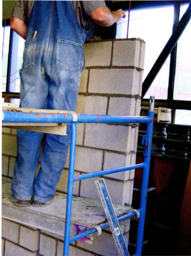
Figure 3.1 Reinforced masonry walls under construction
