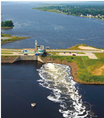
Annapolis Royal Tidal Generating Station (Gielkens 2008).
