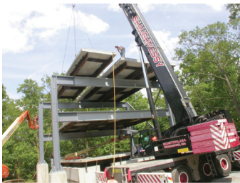
Concrete overpass being placed on steel structure. (ArchDaily 2012)
