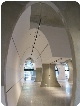
Precast concrete portal frames (BAU n.d.)
