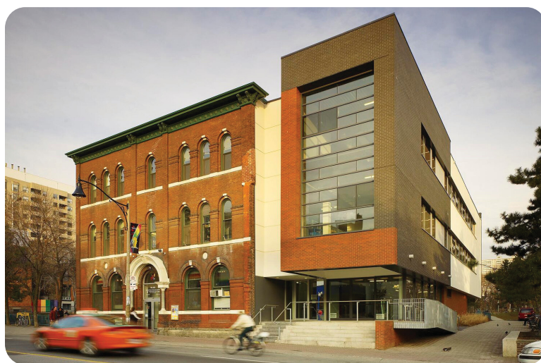
Exterior view of The 519 from Church Street (Kohn Schnier Architects, n.d.)
