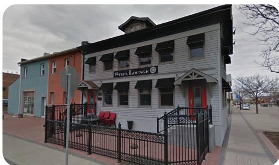
Steel Lounge - Closed 2016 (Google Maps 2016)
