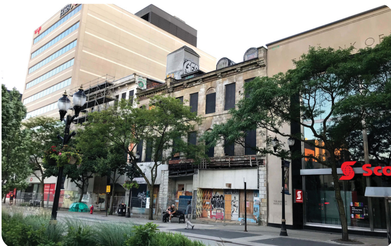
View of the Gore Block in 2022. After sitting vacant for years, the pedestrian life in Gore Park has dwindled
