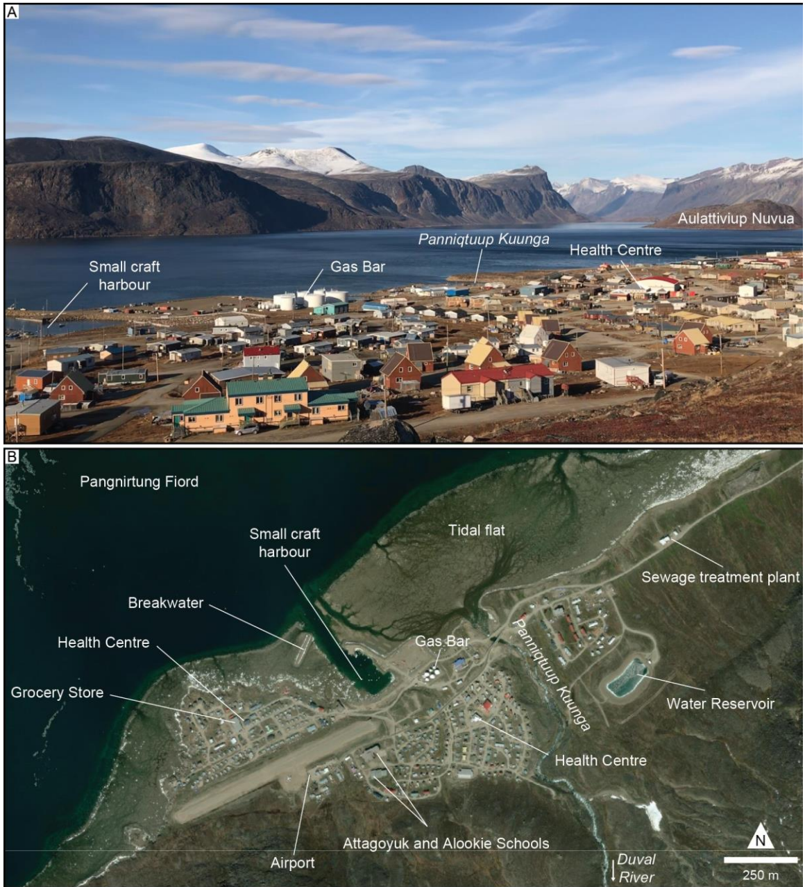
Figure 1.2: a) North view of the hamlet of Pangnirtung (Nunavut). b) Aerial view of the hamlet with key infrastructure labelled. Base map from Maxar Technologies.
