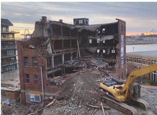
Partially McClary Manufacturing Building, December 2021 (Adam Theriault 2021)
