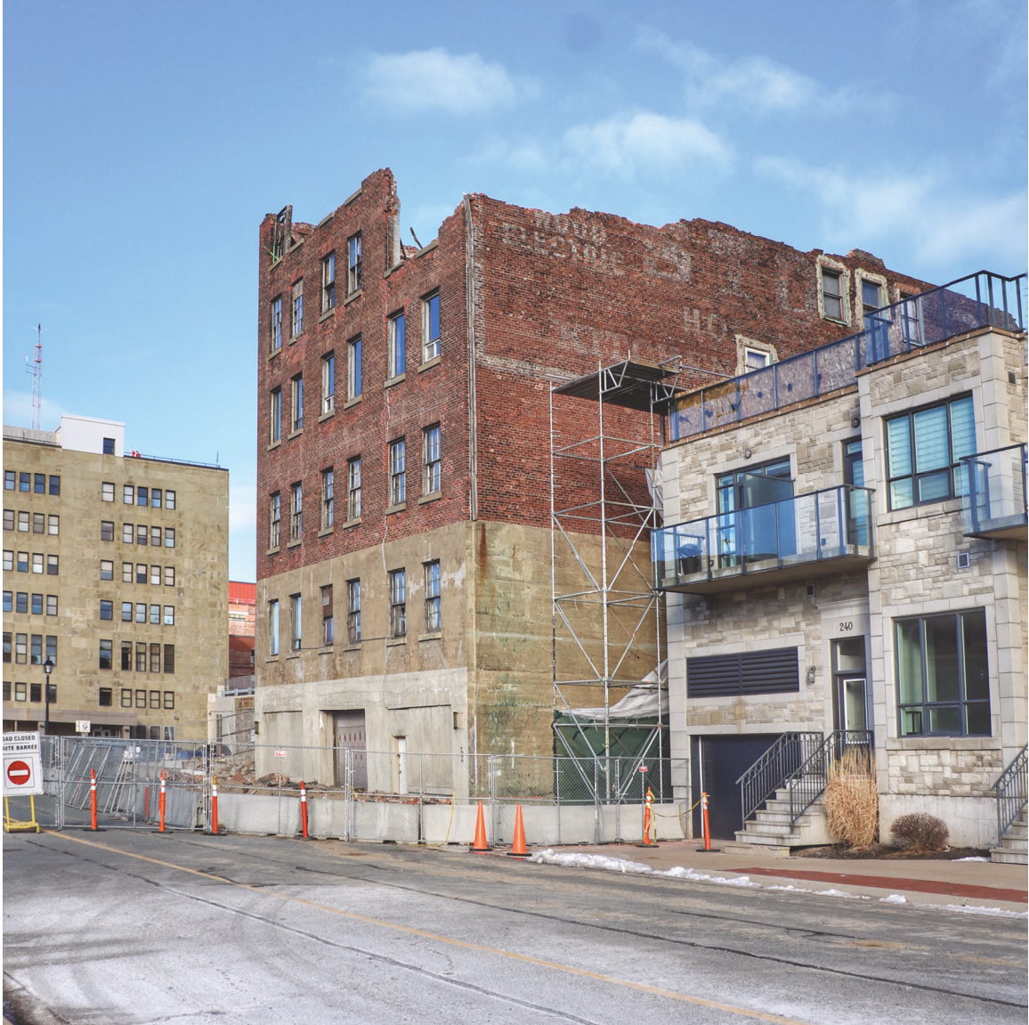
Partially Demolished McClary Manufacturing Building, December 2021
