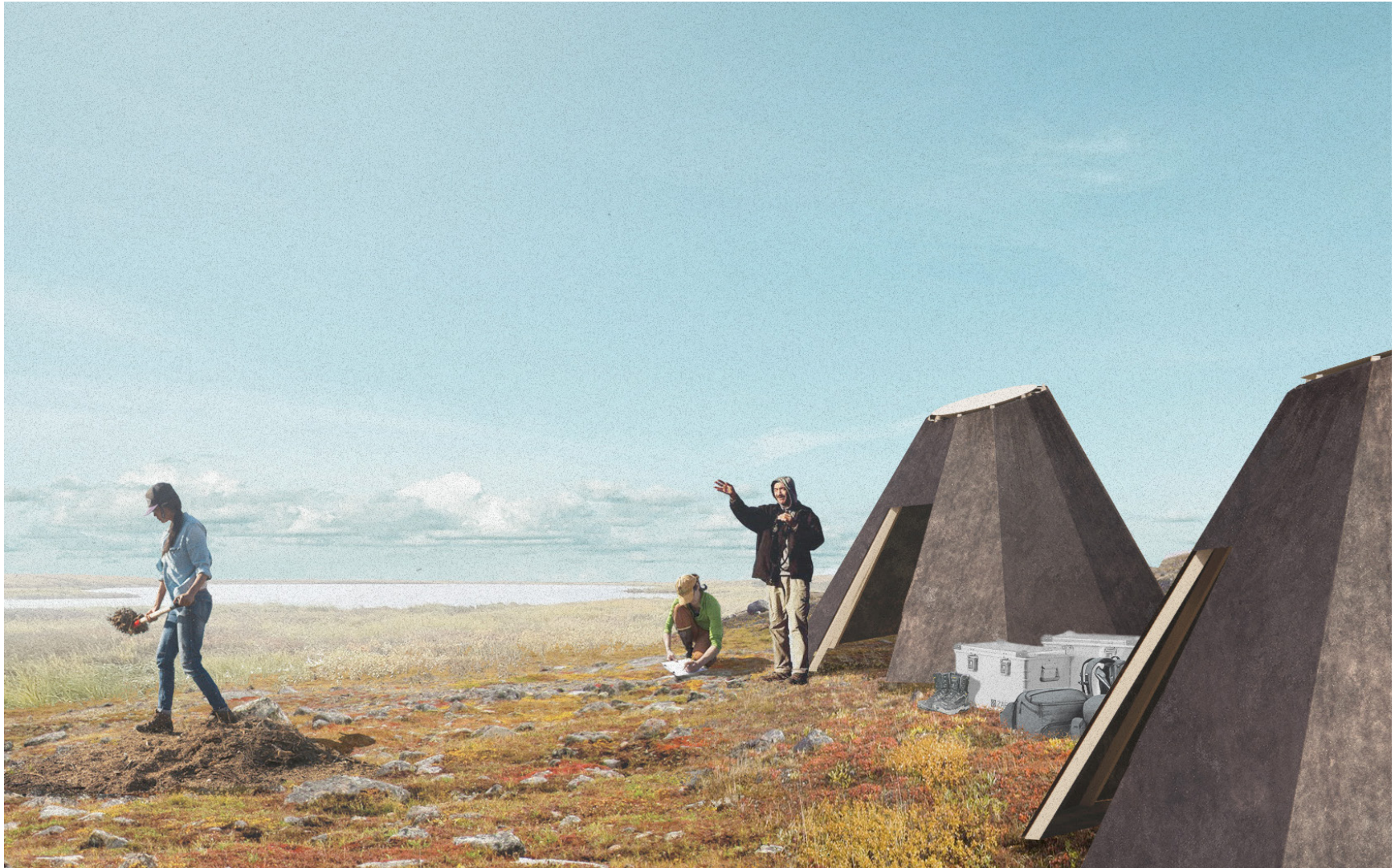
Rendering of the temporary shelters set up at a temporary camp. These camps act as a network with the main research space in Tuktoyaktuk. Materials (small wood members, steel connections, animal hide, solar panel roof) negotiate Indigenous and Western approaches to research.
