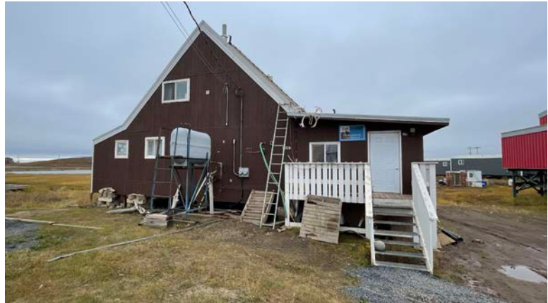
Greenlander building type. Additional side entry with kitchen, bath and bedroom added to the original building.
