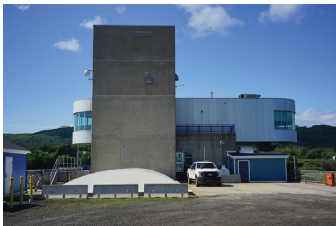
Photographs of Annapolis Royal Generating Station, 2021.
