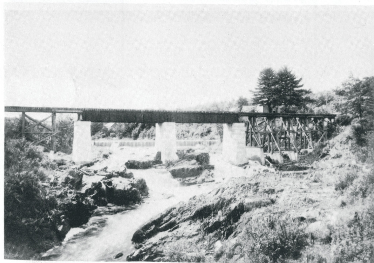
Concrete dam for water power and railroad trestle, Nictaux Falls, Nova Scotia.
