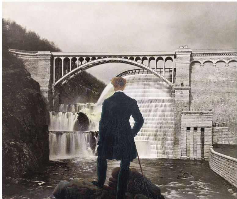
G. V. New Croton Dam. Spillway and ownstream face. April 19, 1912.
