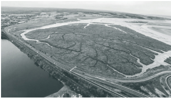
Silt buildup from the Windsor Causeway (Devet 2017)
