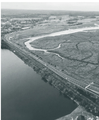
Aerial view of the Avon River Causeway (Devet 2017)
