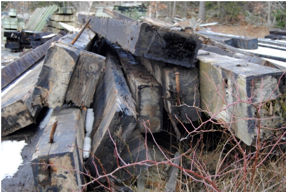
Fig. 6.1. Decommissioned timber girders
