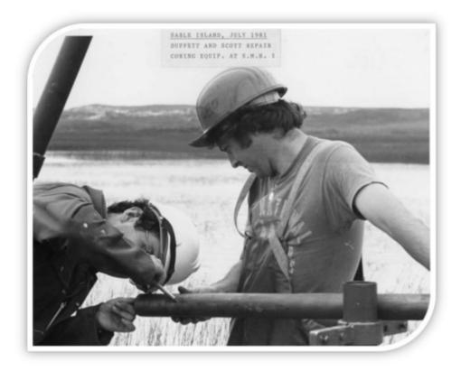
Dave Scott and Tom Duffett repairing equipment and recovering vibracores used in foraminiferal analysis to examine the evolution of Sable Island (July 1981). Scott's research with forams deciphered the record of sea level change affecting Sable Island.
