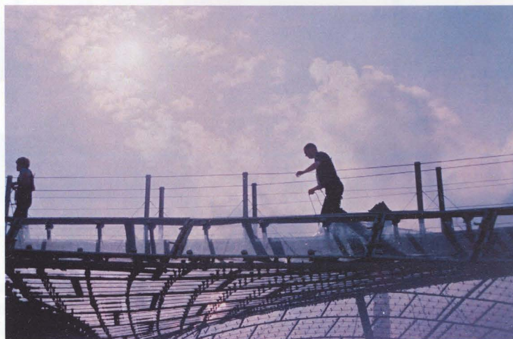
Tours of the canopy roof of the Olympic stadium in Munich, Germany
