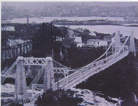
Photograph of the former Reversing Falls cable suspension bridge from (Schuyler 1984, 75)
