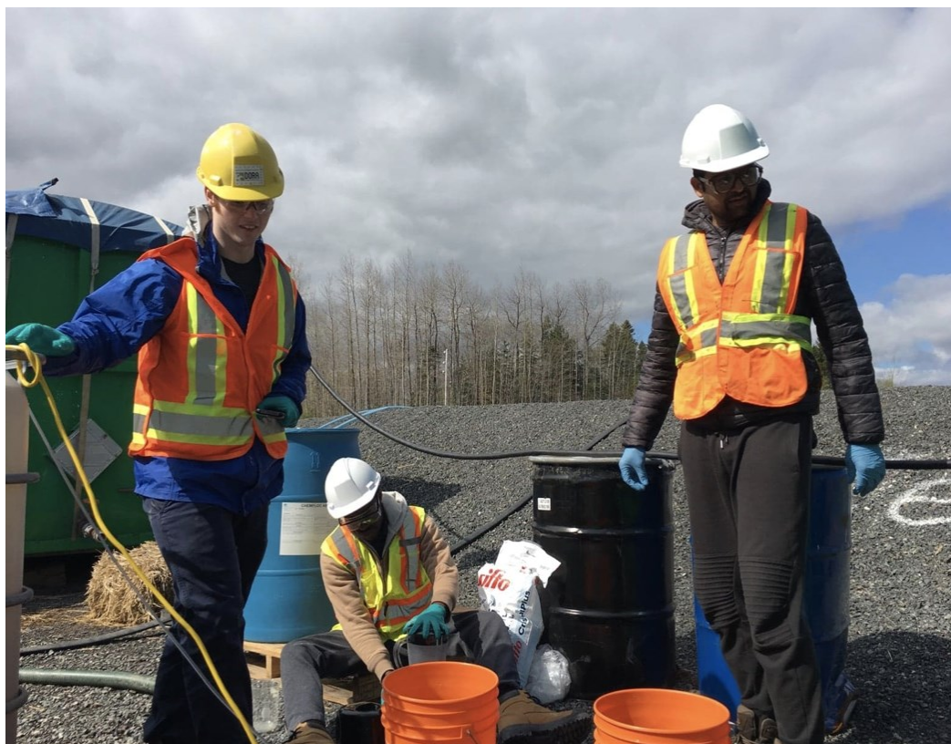
Figure 1. Group members wore protective equipment when onsite at Boat Harbour. Geotube® filtrate was collected when onsite.
