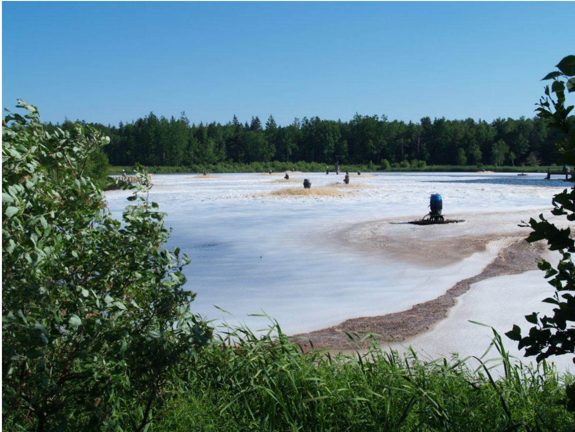
Figure 7. Aeration Stabilization Basin Located at Boat Harbour (Baxter, 2019).
