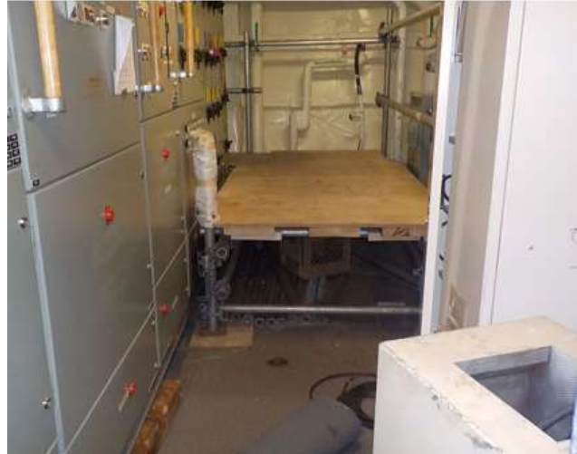
Figure 5: Staging often excludes other work in the same compartment.
