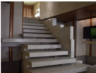
Observations between stair and intentional gap to reveal metal connections
