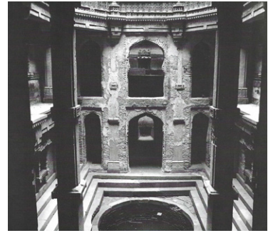
Facing north at Level -4. (Livingston 2002, 99)
