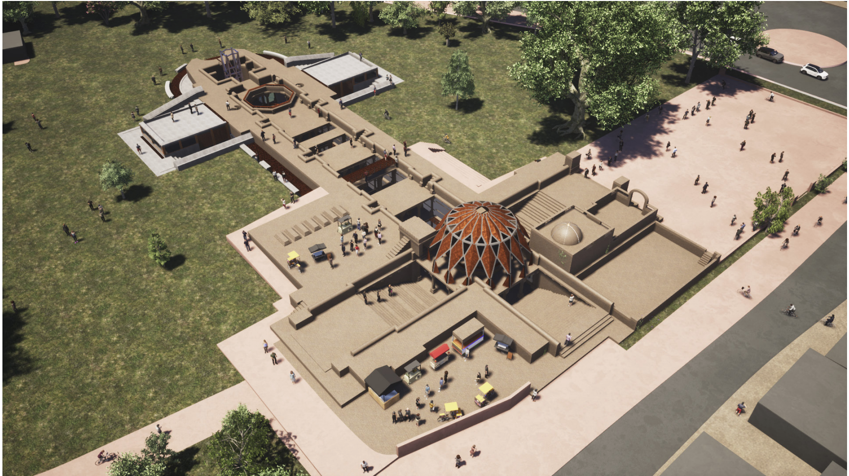
Drawing showing all above ground architectural interventions such as: the dome, bridge, computer lab, multi-use space, elevator that takes one into the subterranean spaces, and the water fountain
