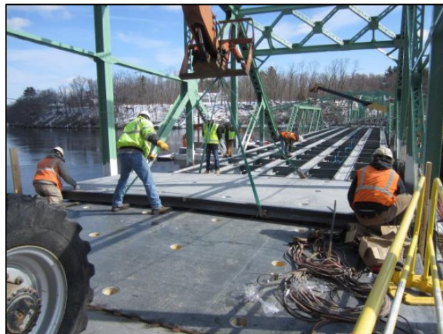
Figure 2-3 Picture of all-FRP panels being installed for a re-decking project (Loff 2015)
