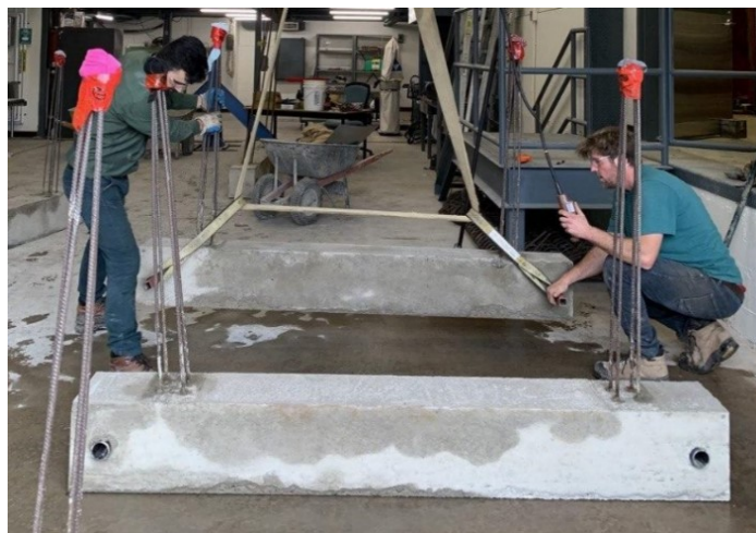
Figure 3.9 Air curing of RC base beams
