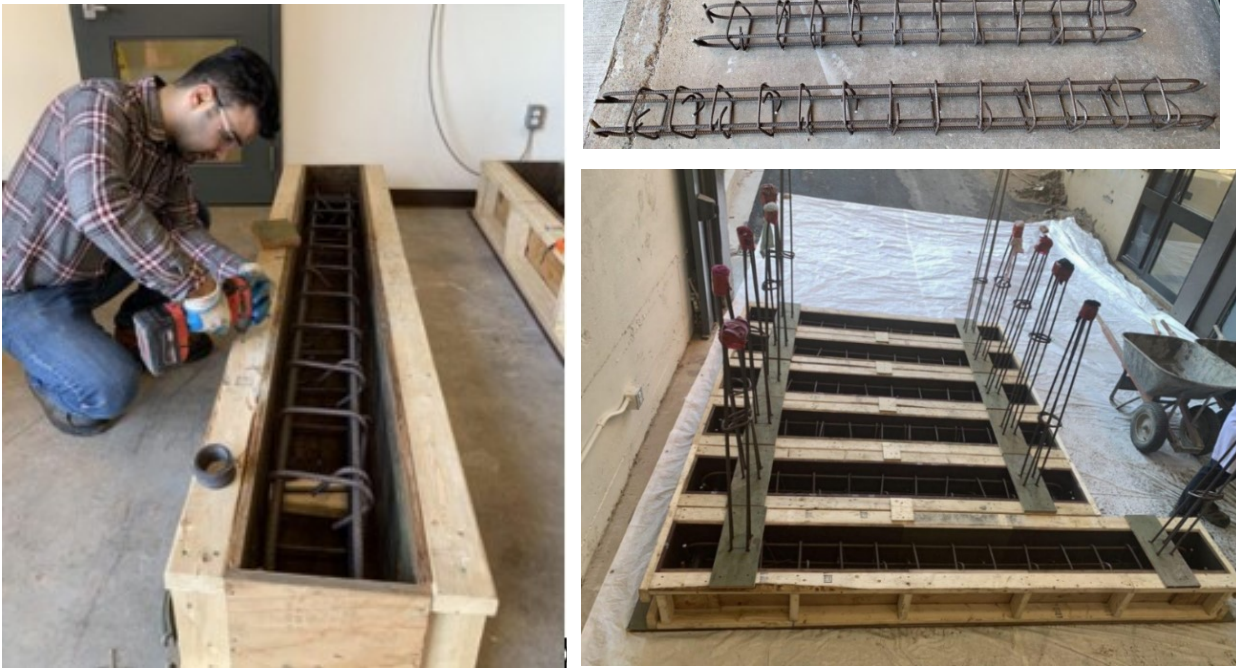
Figure 3.6 Construction of base beam concrete formwork and rebar cage
