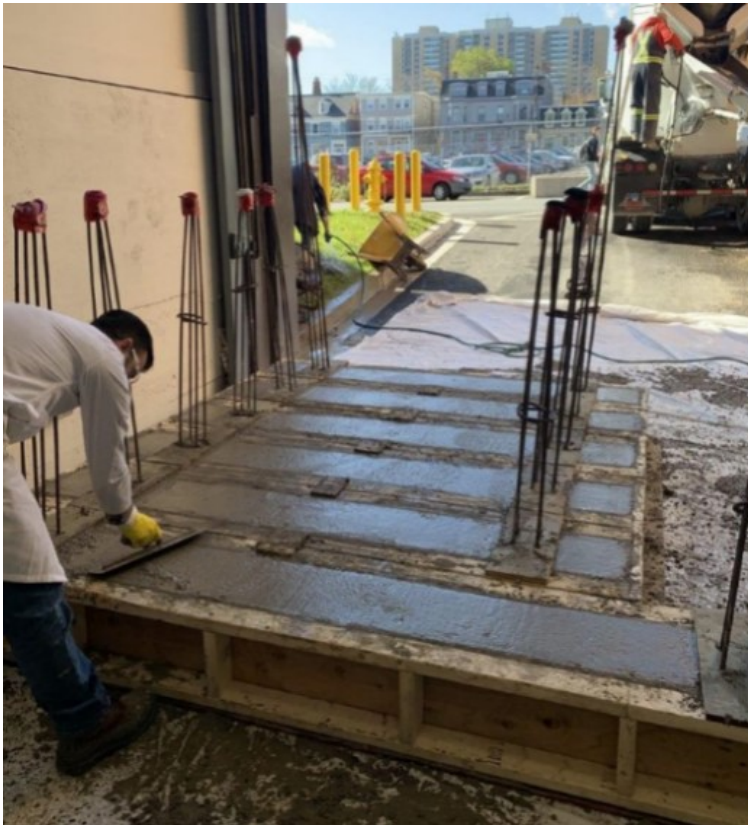
(b) Smoothing concrete surface
