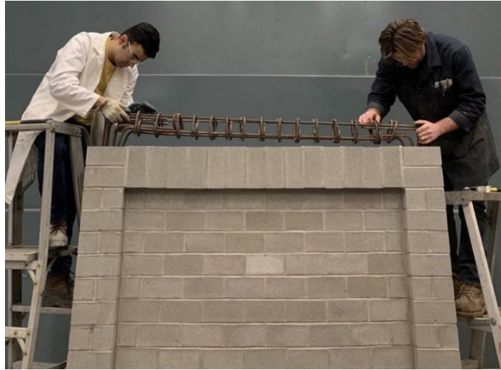
(b) Positioning top beam cage
