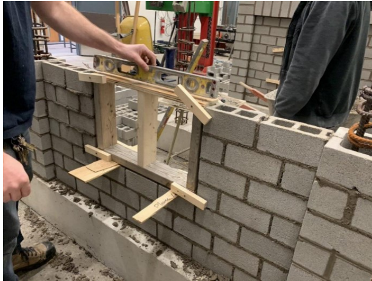
Figure 3.14 The shoring system to form a window opening
