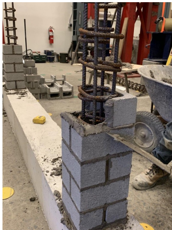
Figure 3.12 Applying mortar to bed joint and head joint
