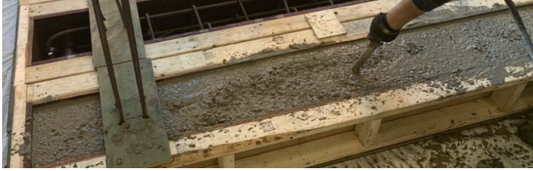
(a) Concrete vibration
