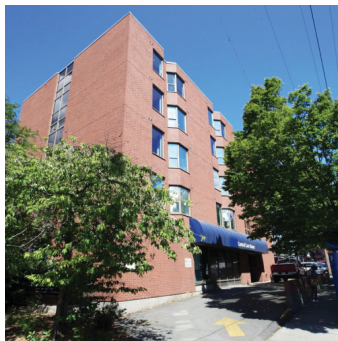
Facade of JSC; photograph Darren Stone (Petrescu 2016)
