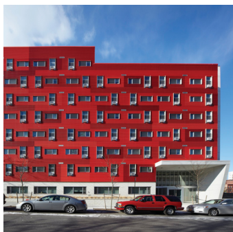
Navy Green, Brooklyn; photograph by Tom Powel Imaging (Architecture in Formation and Curtis + Ginsberg Architects 2015)
