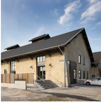
Facade of H17 with staircase and ramp leading to the corner entrance (PLH Arkitekter 2016).
