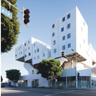
Star Apartments, LA; photograph by Iwan Baan (Michael Maltzan Architecture 2014)
