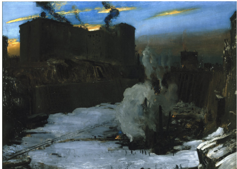
George Bellows, Pennsylvania Station Excavation , 1909 (Pauli 2003, 18)
