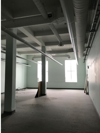
Interior of original concrete building
