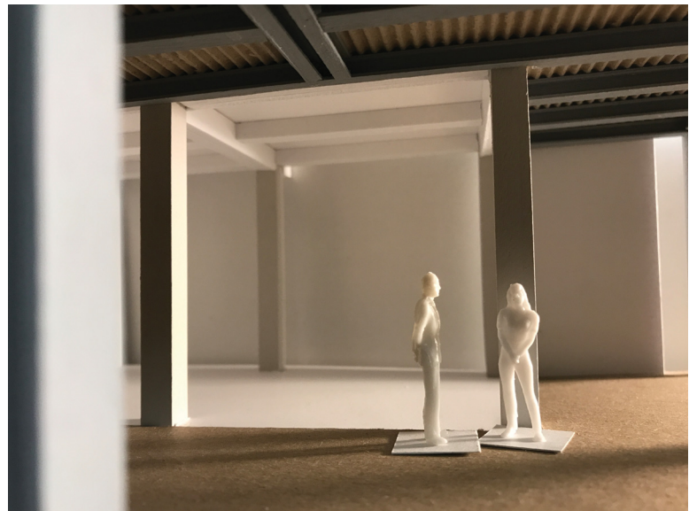
Existing interior - interface between original concrete and steel addition.
