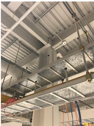
Interior of steel addition
