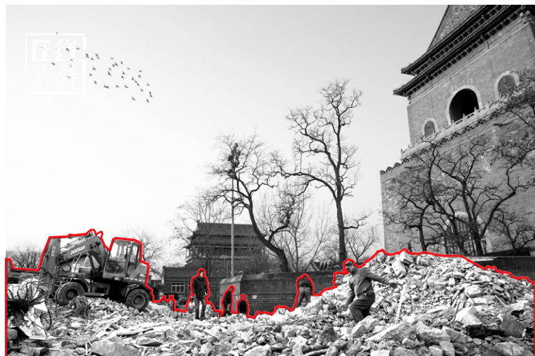
Demolition of Siheyuan in Beijing, photograph by Zhang Jie (Zhang J. 2018)
