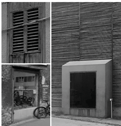
Figure 60 (top left): Vernacular wooden lamella haybarn element which appears to be re-appropriated in Zumthor's enclosure system
