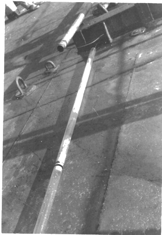
b. Setting up of core liner.
