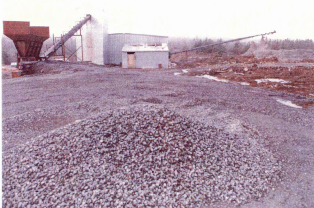
Figure 4.1b This picture shows the new mill structure while it was in use during the 1980s. Tailings are actively being discharged near the right side of this image (photo courtesy of Nova Scotia Department of Natural Resources).
