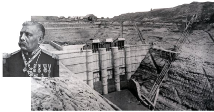
1897 Dam gates of the Grand Canal and drain.
