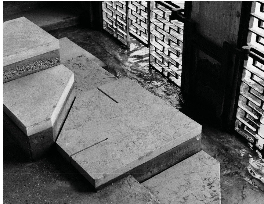
Water entering into the entrance of the Plazzo Querini Stampalia, 2016; photograph.
