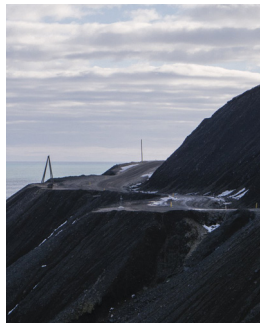
Vulnerability to rockfalls, slope failure and ground flows.
