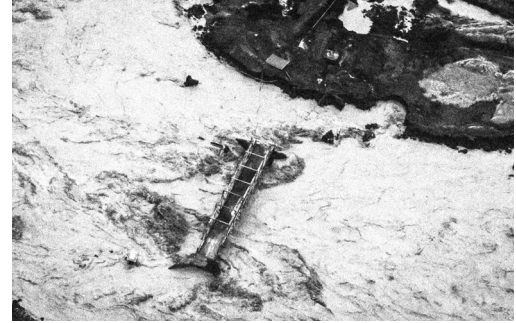
Washed out roads divert the flow of flood water to alleviate pressure on bridges to protect the infrastructure.
