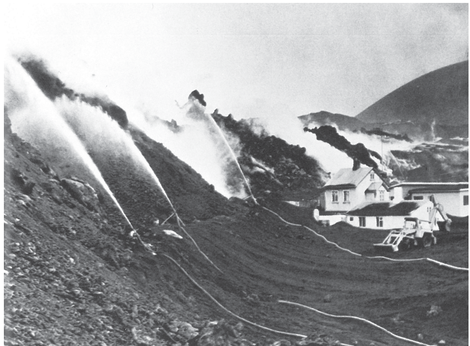
Water sprayed in efforts to solidify the lava flow and protect the town and harbour. Þorleifur Einarsson, ( Heimaey Utbruddet , 1973)
