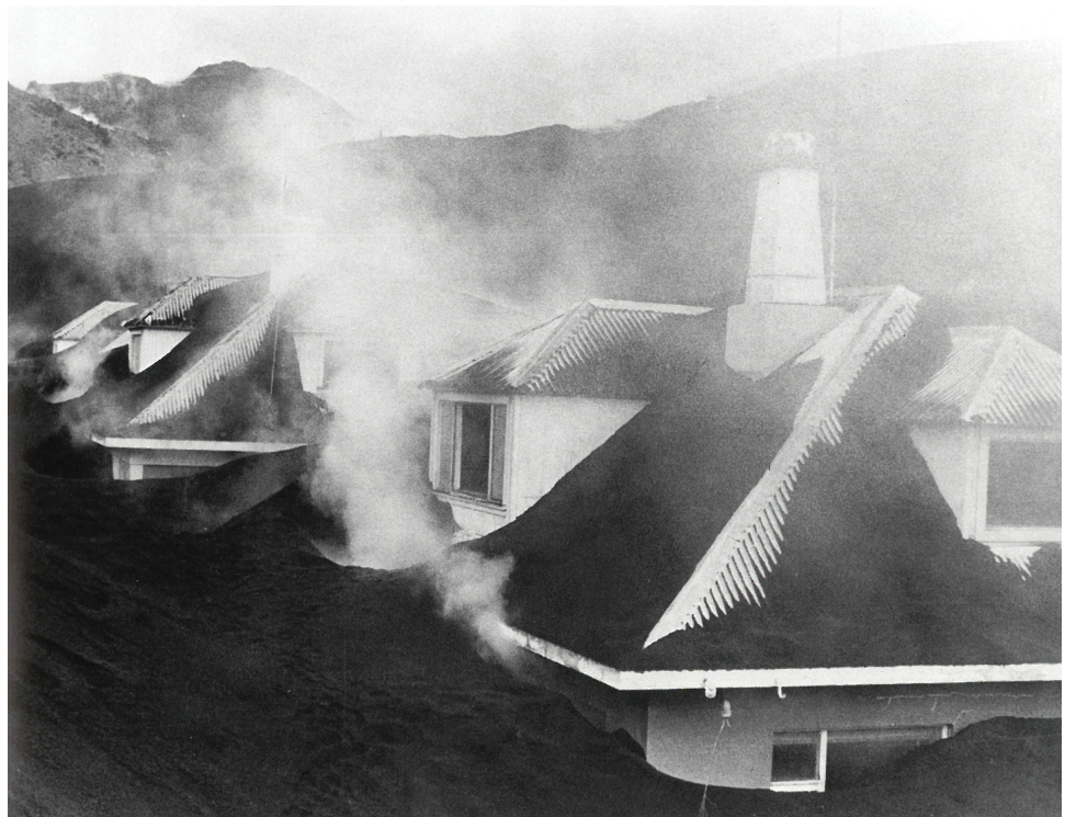
Ash-lined street in Heimaey. Many homes succumbed to the heat and weight of the falling tephra. Þorleifur Einarsson, ( Heimaey Utbruddet , 1973)
