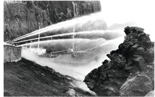
Sea water sprayed on encroaching lava flows to collect the material, cooling and solidifying.
