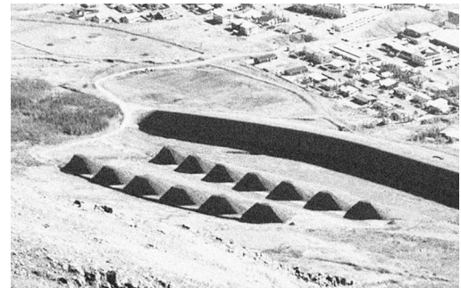
Avalanche dams and barriers disperse flowing earth and snow.
