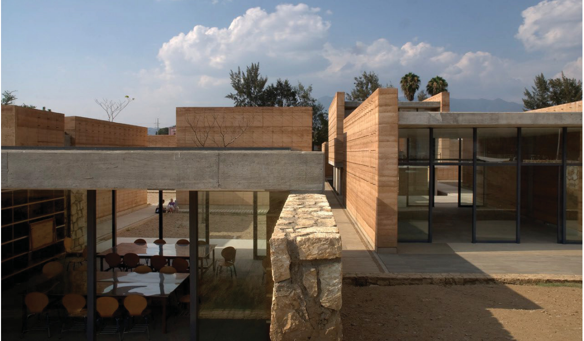
Figure 56 is a photographs of the School of Visual Arts. The image shows a contrast between rammed earth and stone walls. Photograph by Luis Gordo and Rafael Carrillo.
