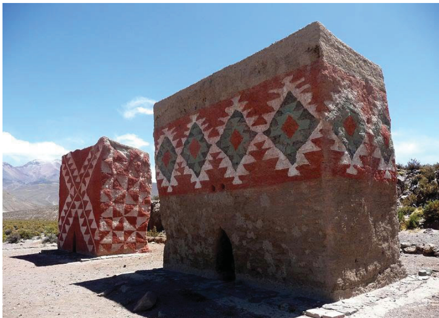
Figure 45 shows the construction of the Chulpas, with soil that colours the building. Photograph by Tierradevientos.
