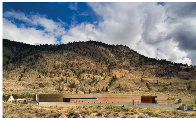
Figure 52 is a photograph of the NK'Mip Desert Cultural Centre. It shows the expression of rammed earth with the blending into the landscape of Osoyoos. Photograph by Nic Lehoux Photography.
