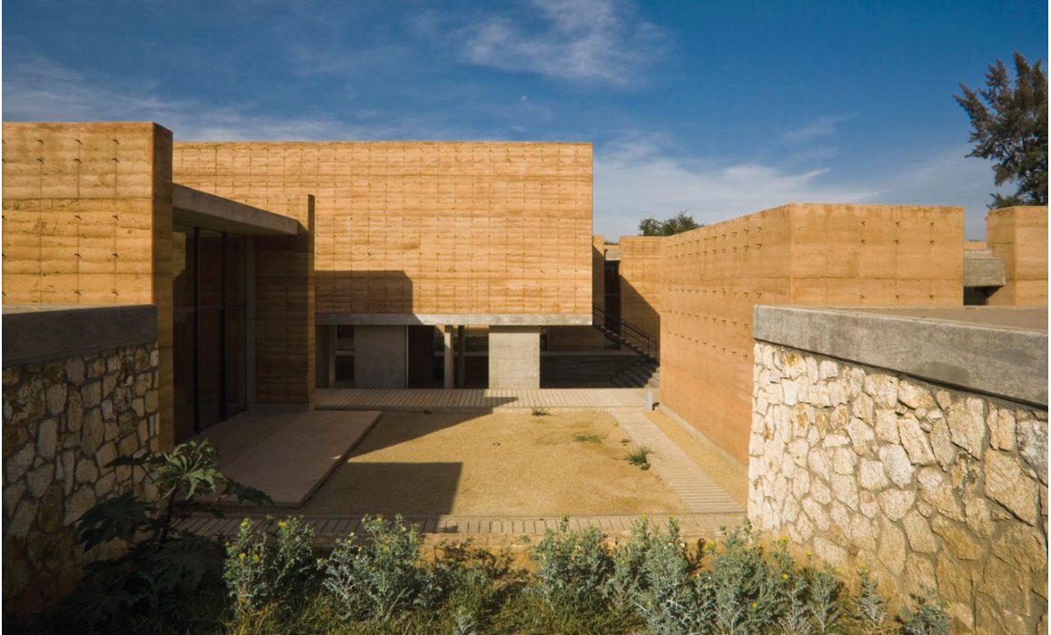
Figure 55 shows the School of Visual Arts. The image shows a contrast between rammed earth and stone walls. Photograph by Luis Gordo and Rafael Carrillo.
