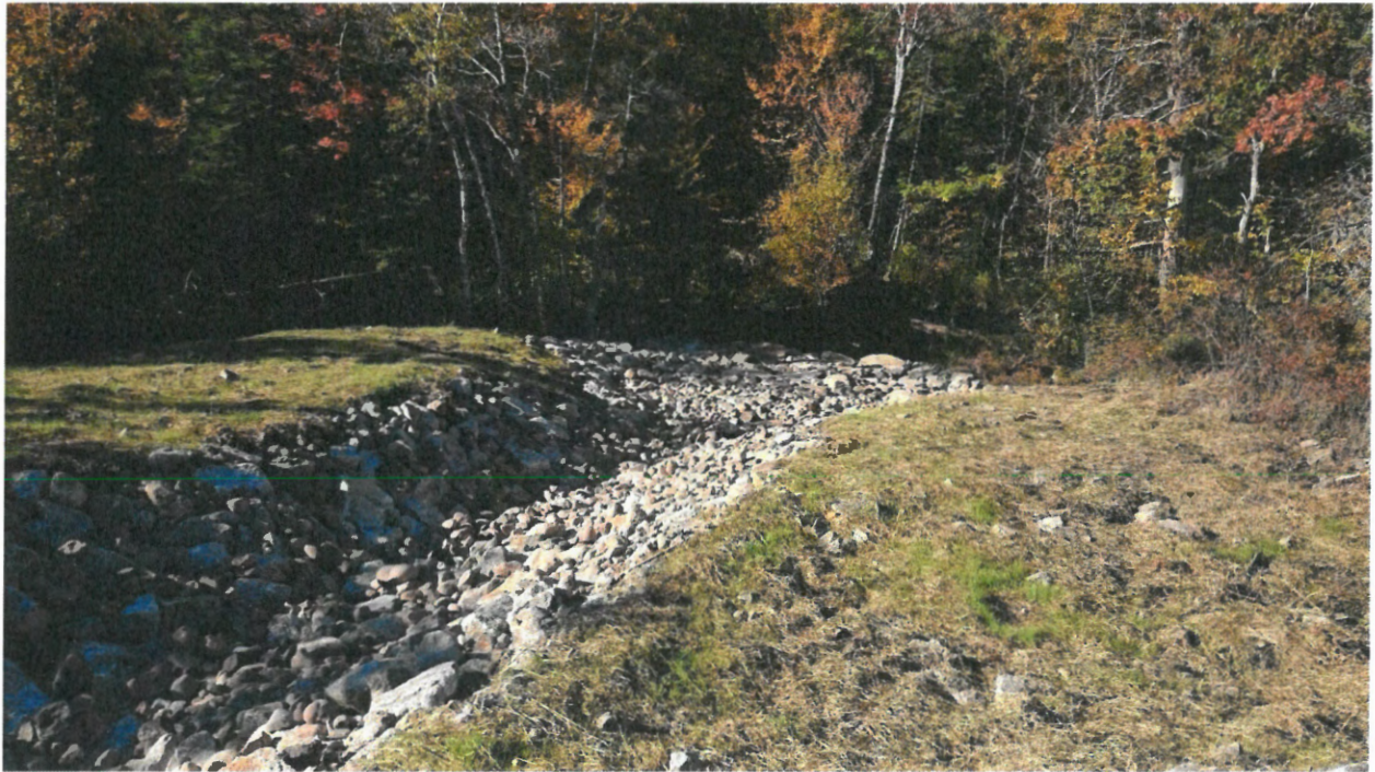
Figure 16: (Top) Standing near McIntosh Run at Governor's Brook Development; Storm water drainage channel directly into McIntosh Run. (Bottom) Storm Drainage channel into McIntosh Run.
