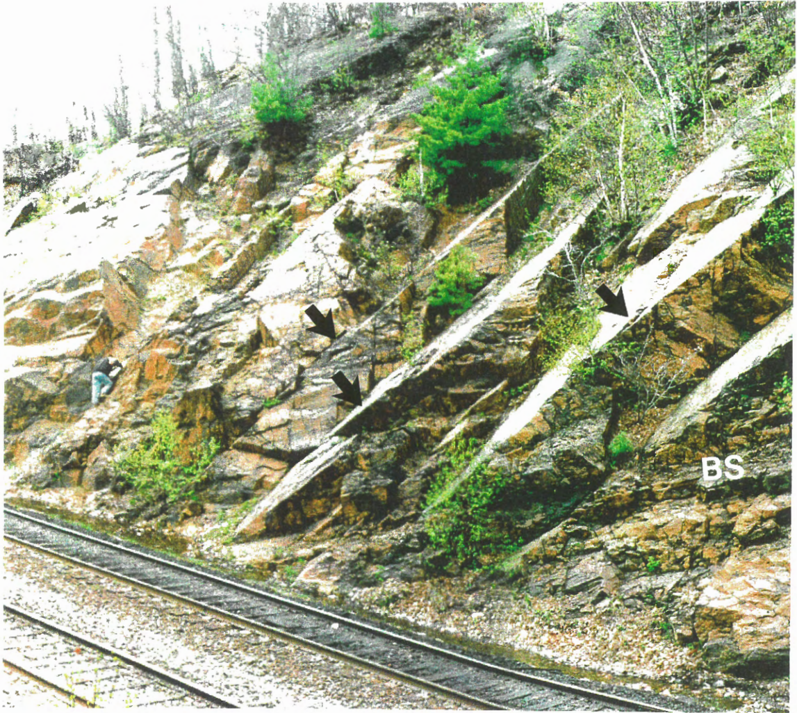
Figure 2.16: Photograph of well developed, regularly spaced lateral ramp movement horizons, indicated by arrows, exposed along the railway tracks west of Tower Road (see Fig. 2.2 for location). BS = bedding surface, which strikes roughly parallel to the photograph and dips out of the photograph.
