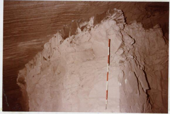
PLATE IV.A.9. "Ridge and furrow" moulds on back sandstone, caused by deposition over slump folded and truncated mudstone beds, (visible at top of wall), 2-5-4 drift. (ranging rod = 2 m).
