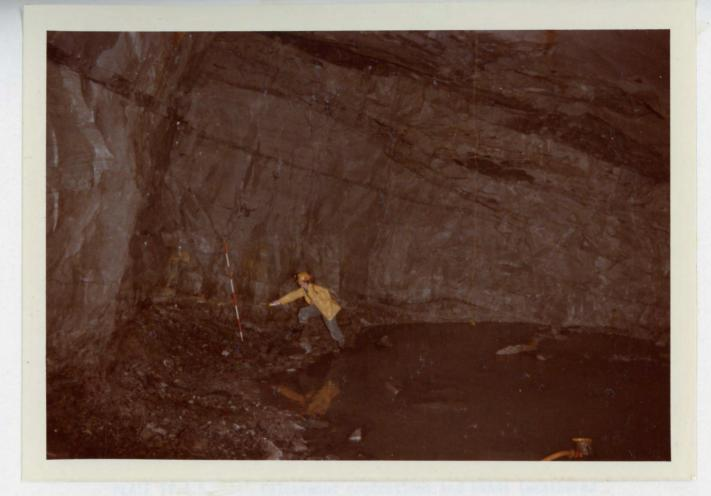
PLATE IV.A.4. Typical sandstone host rock - Working face No 3 decline. (ranging rod = 2 m)
