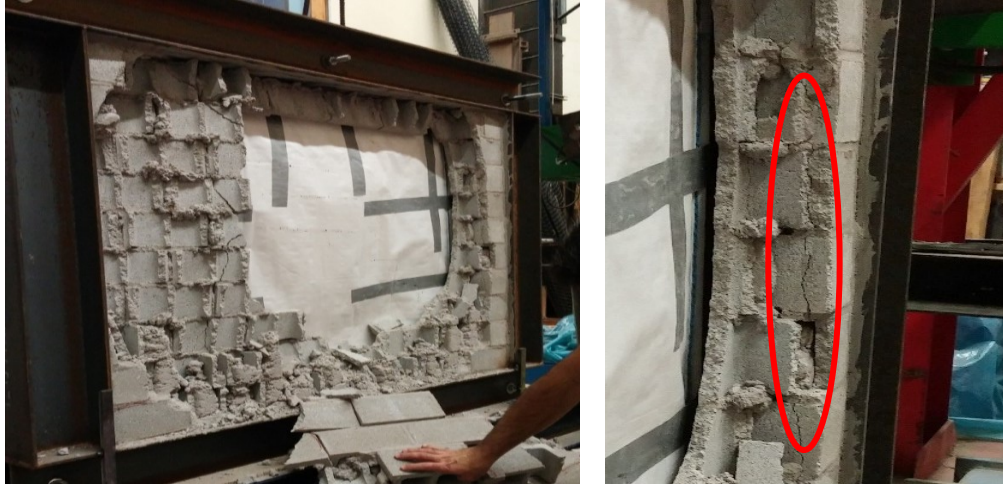
Figure 4.7 Faceshell separation due to web shear failure on specimen IF-S-FS
