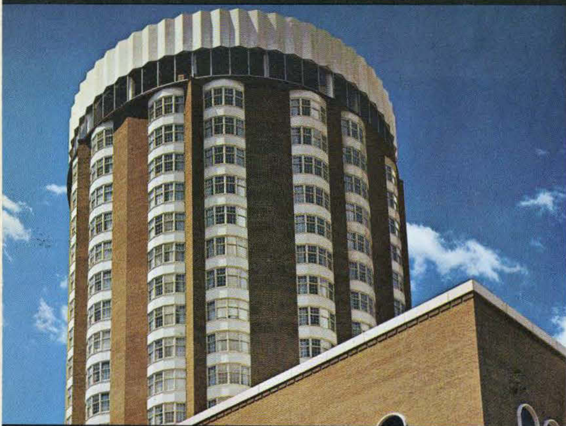
Architect: Rasche-Schroeder-Spransy and Associates • Contractor: Hunzinger Construction
