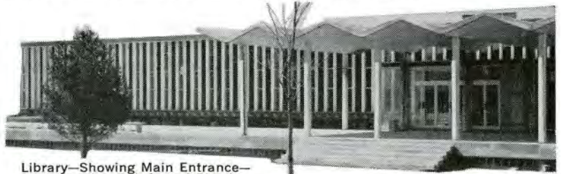
Library—Showing Main Entrance—Incorporating Reinforced Plastic Fins and Panels.
