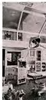
Operating Room Toronto General Hospital Architects Mathers & Haldenby
