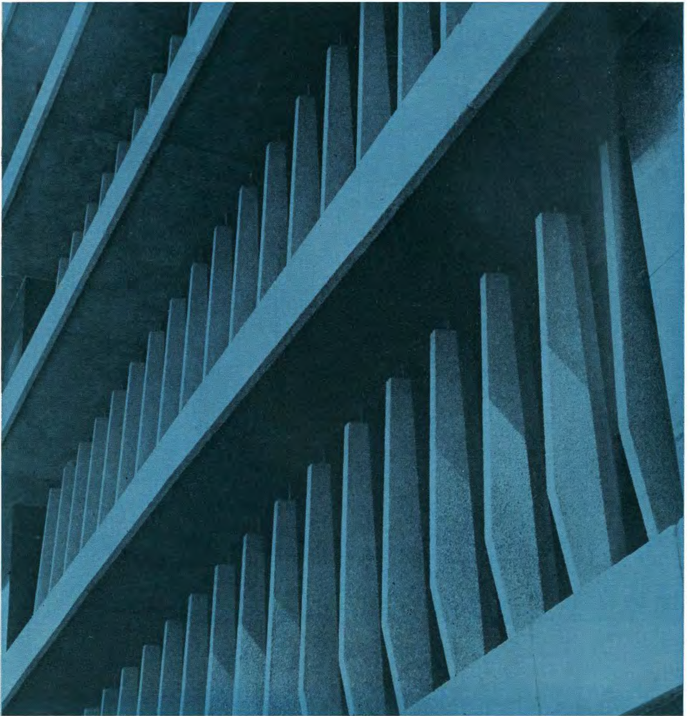
Architect: Maxwell Miller (Simpson's) Ltd. • General Contractor: Pigott Construction Ltd. • Panels: Precast by Pre-Con Ltd.
